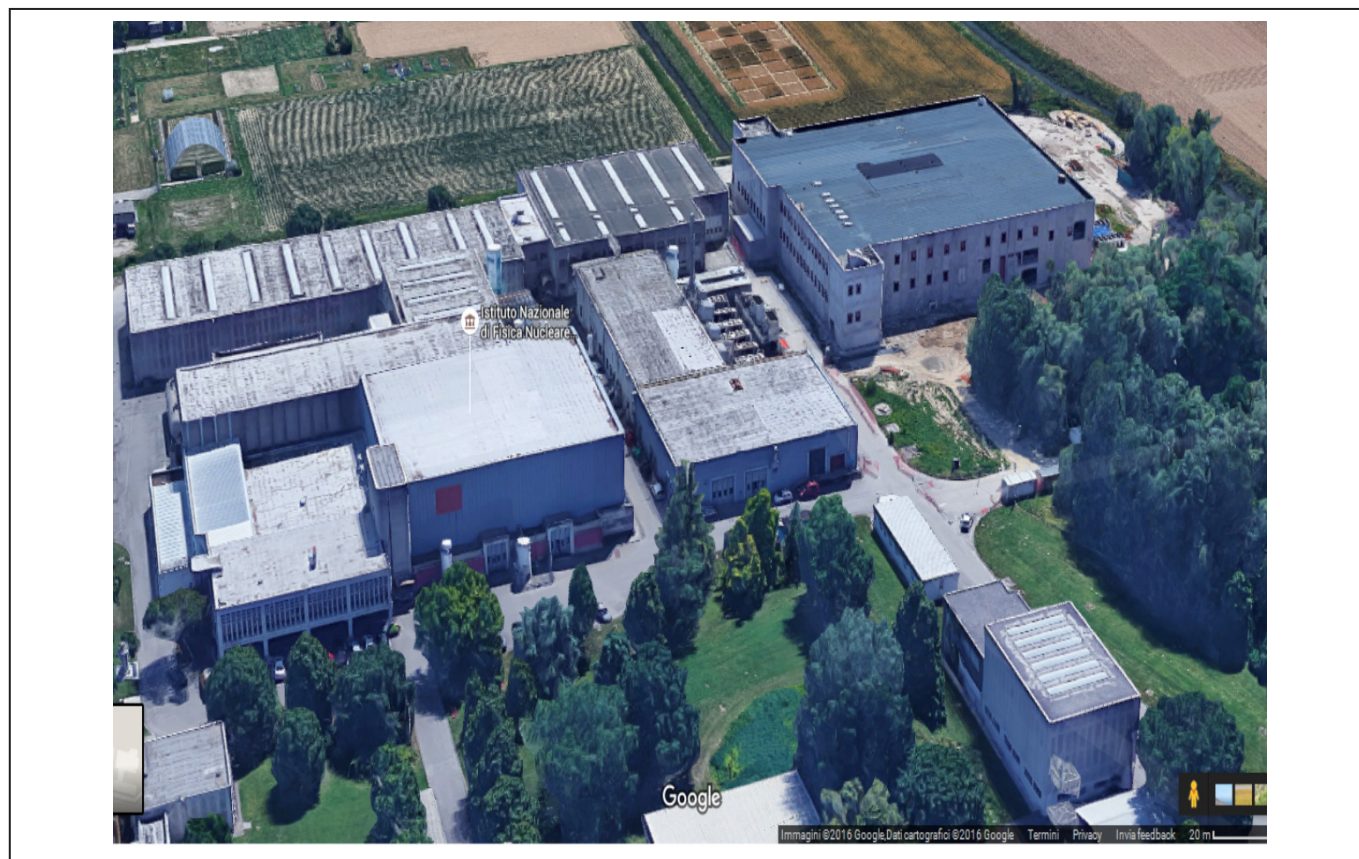
Figure 1. View of the new SPES building (on the upper right) and of the old TANDEM _ALPI complex (on the left).
